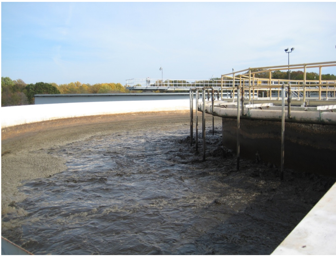
Biosolids Thickener Tank
